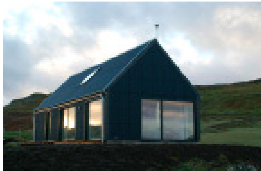
Below The Black House, Clashnessie, north-west Scotland (2009). Corrugated fibre cement-clad house with large kitchen/dining/living room, bedroom and bathroom on the ground floor, with a gallery and sleeping loft above. Sliding doors open onto a deck overlooking the beach, with a large framed view west out to sea. The building complements existing ones in the village, which include stone and corrugated metal sheds. (ph: MAF).
