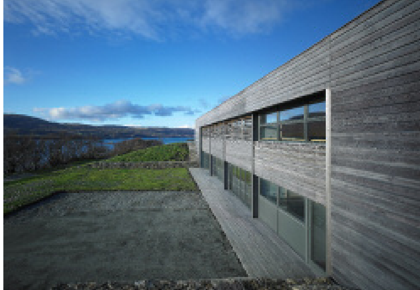
Above The larch-clad south-facing elevation of the community hall incorporates sliding shutters and glazing to the ground floor and fixed lights and sliding shutters above, protected by fixed solar shading.
